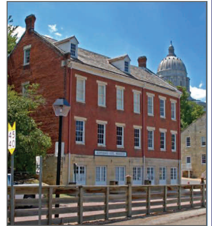
Current picture of the historic Union Hotel locating at Jefferson Landing. It currently serves as the Amtrak Train Station.
