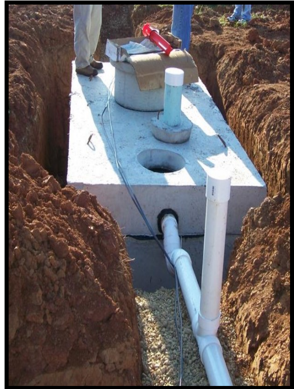
Installation of a 1,000 gallon concrete septic tank.
