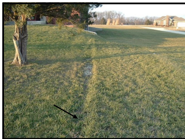
MALFUNCTIONING curtain drain. Grass has been allowed to cover most of the gravel; water is not diverted but flows freely downhill.
