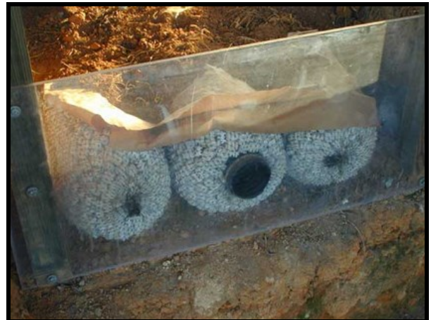
Perforated flexible 4" inch pipe (Expanded Polystyrene Bundles).
