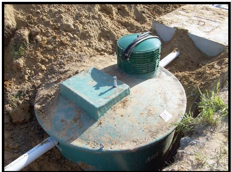
Installation of an aeration treatment unit.
