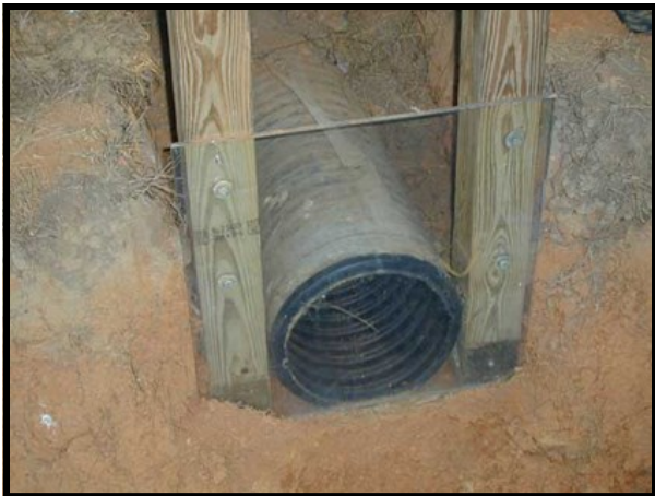
Filter wrapped 10" inch perforated corrugated pipe.
