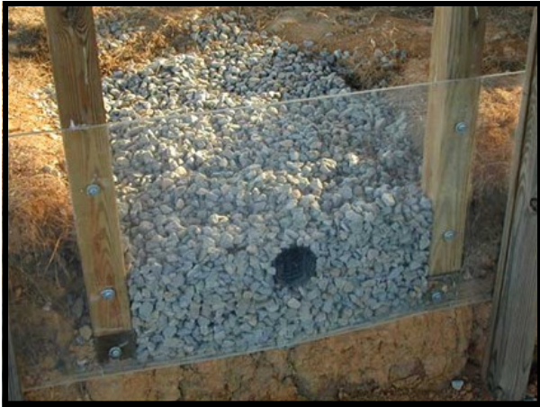
Conventional gravel trench with 4" inch perforated pipe.
