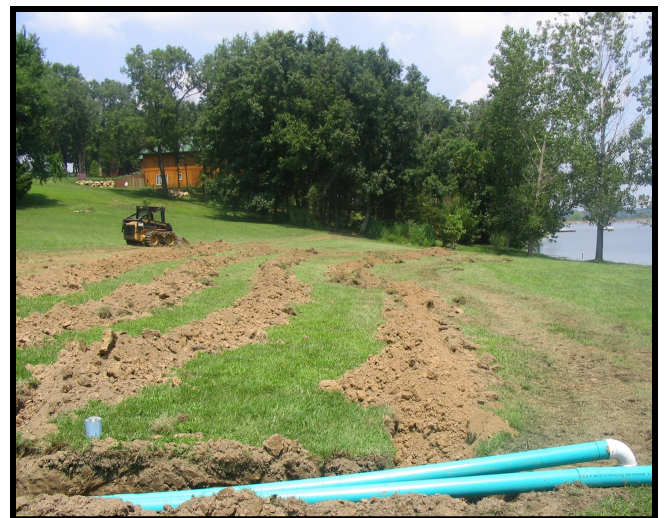
Dispersal trenches installed on contour.
